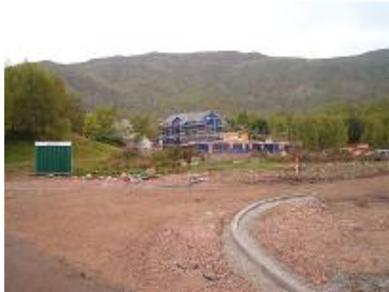
Staff Block under Construction
